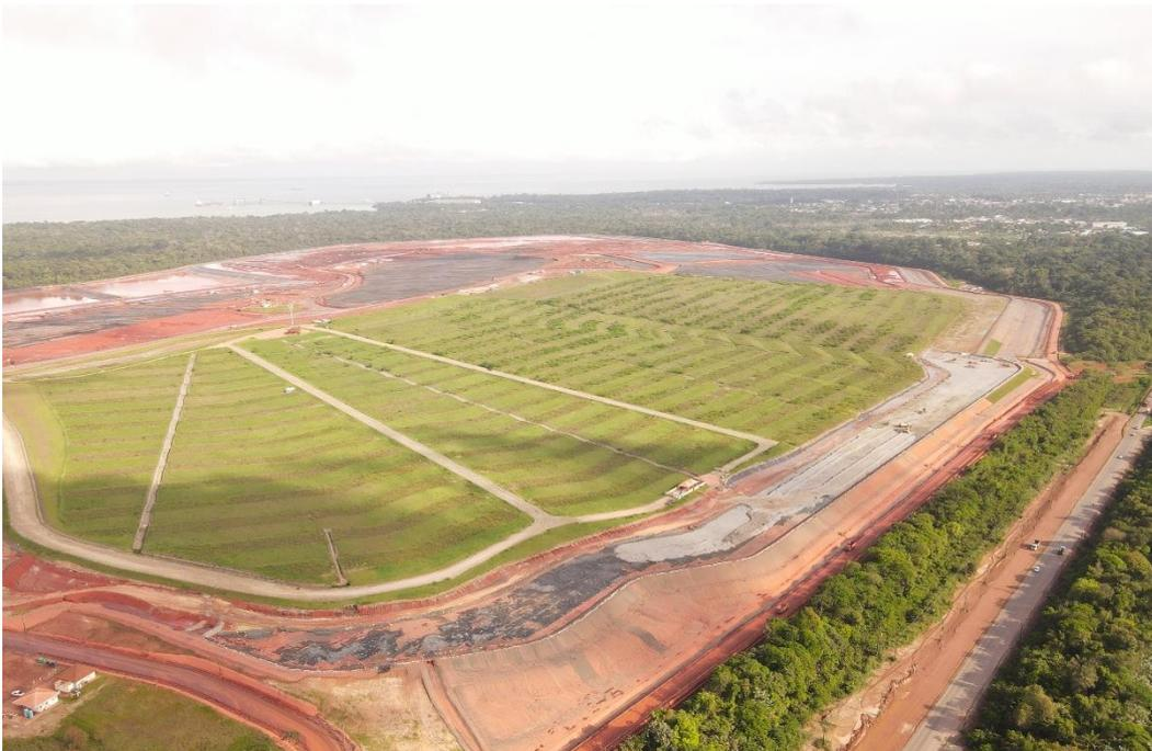
The closure is divided in 11 strips of rehabilitation. The strips 2, 3 and 4 have been rehabilitated, and represent approximately 60 ha. The design considers cap and store the filtered residue with cover systems consisting of HDPE geomembrane to lining the stored residue, covered by a densified soil, and revegetation of the surface.
